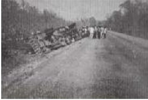
Steep side of this earthen “V” drain may have caused the vehicle to overturn.
