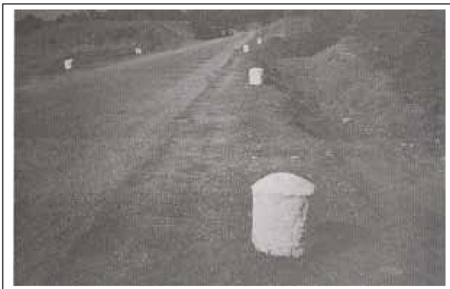
*Figure 4: Earth-filled bitumen drum as delineating device*
