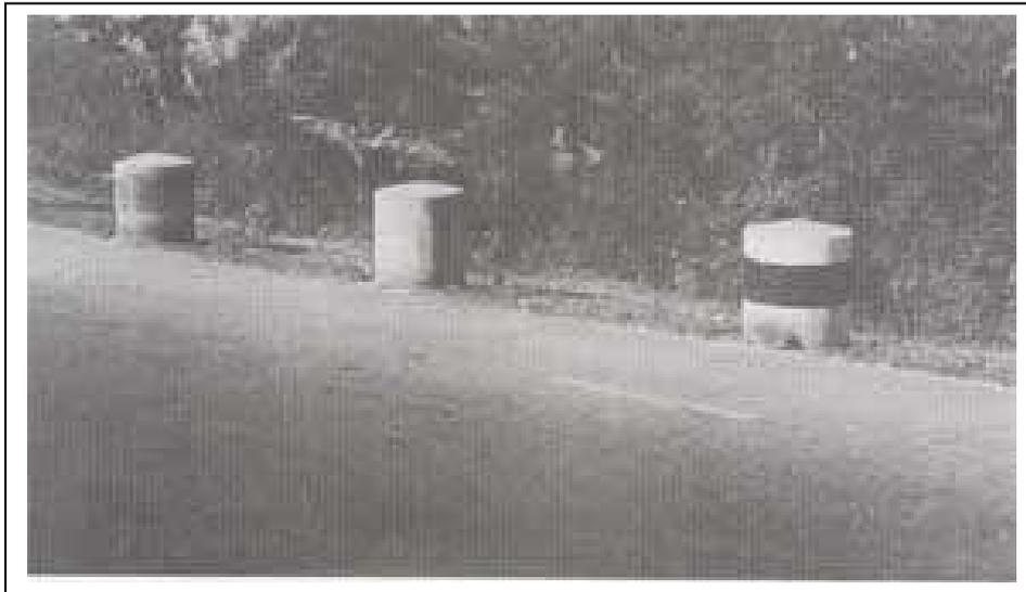
*Fig. 3: Confidence blocks of concrete (drum)*
