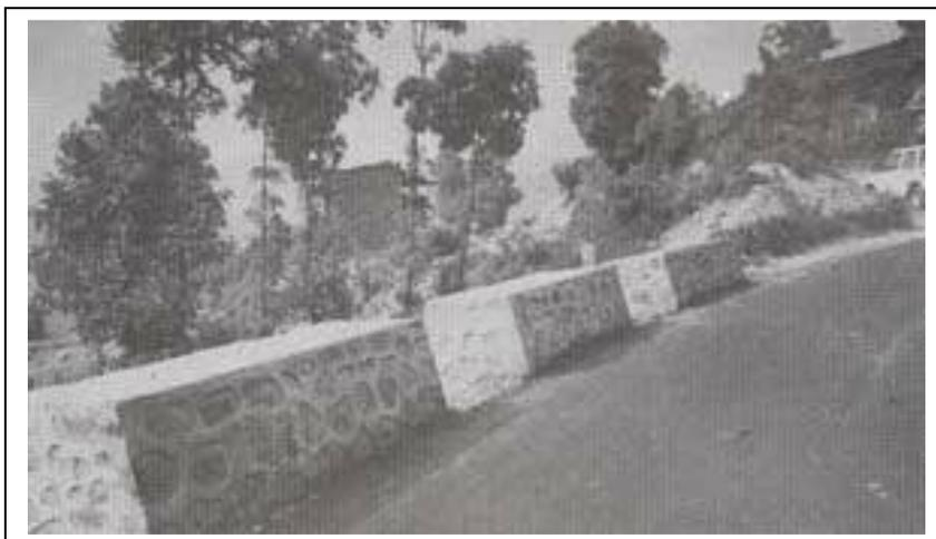
Fig. 4: Plum concrete barrier blocks
