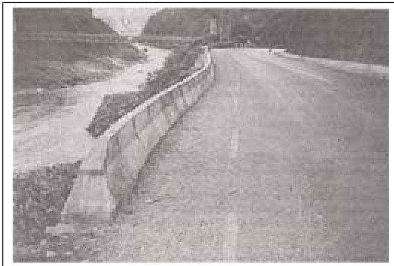
Fig. 6: Pre-stressed RCC barrier
