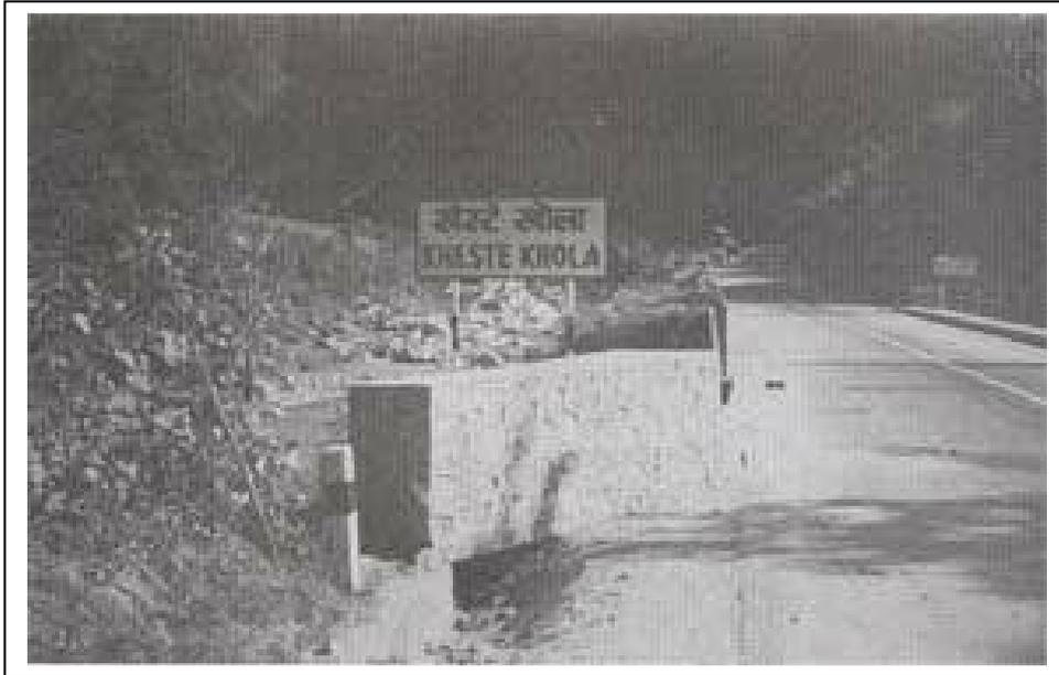
Fig. 3: Random rubble masonry barrier
